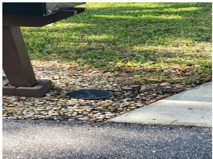
ATRIUM DRAIN LEADING TO STREET
