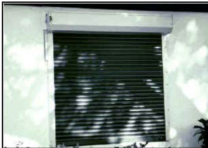
HURRICANE SHUTTER, CLOSED
