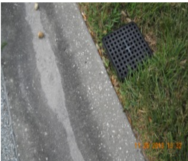
COURTYARD DRAIN LEADING TO STREET
