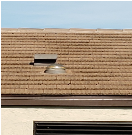
SOLAR TUBE SKYLIGHT
